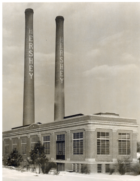
Hershey powerhouse, ca. 1924-1940
